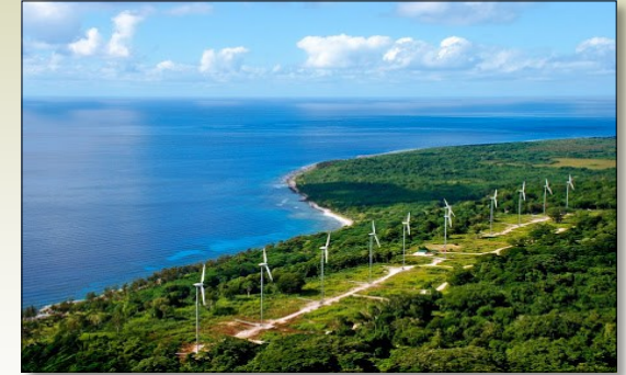
Windmill used for producing electricity for lighting at Devils Point, Efate.
