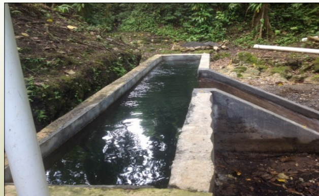
A mini hydro system used to produce electricity power in a village in Vanuatu.
